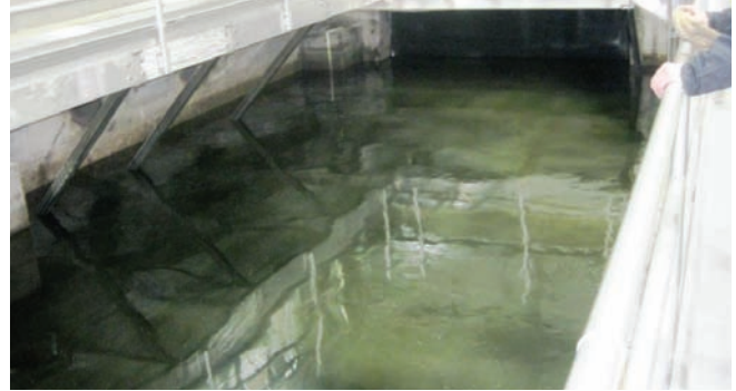
Figure 2. High TSS Secondary Effluent during Performance Testing
