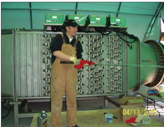
Photo 1: Installation of UV Lamp Sleeves in Catskill/Delaware UV Unit
