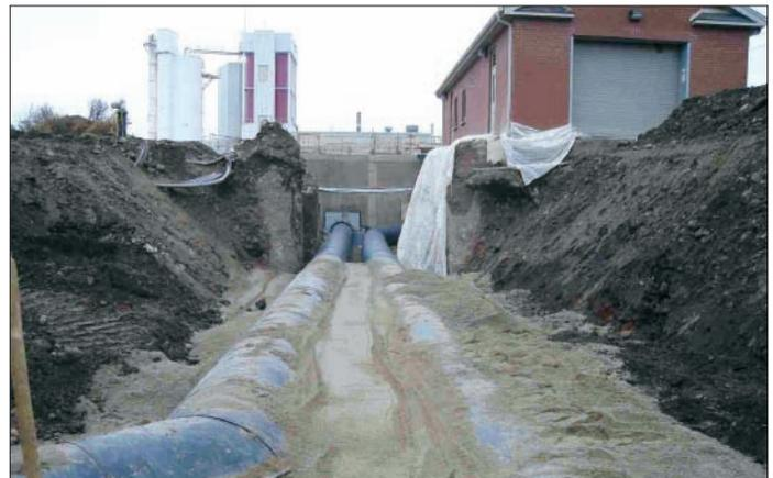
**Figure 7.** A construction photo of the interconnecting piping being installed from the new UV facility to the Valve Chamber where incoming flow is directed throughout the Woods site.
