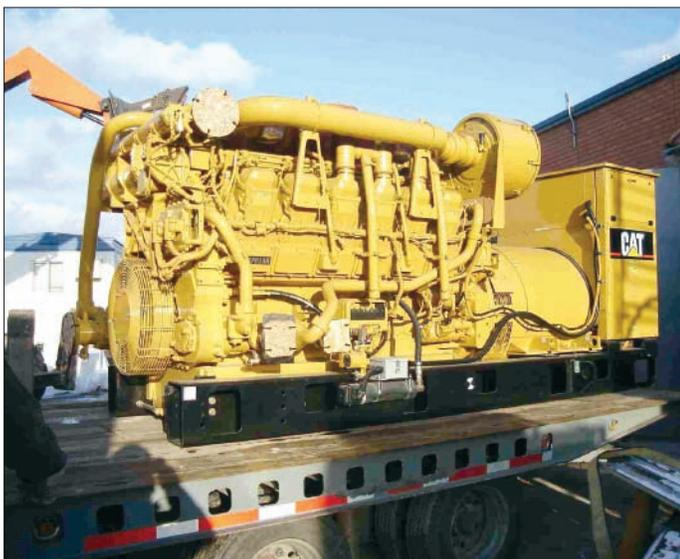
**Figure 6.** The generator set being rigged into the main FMWoods Building
