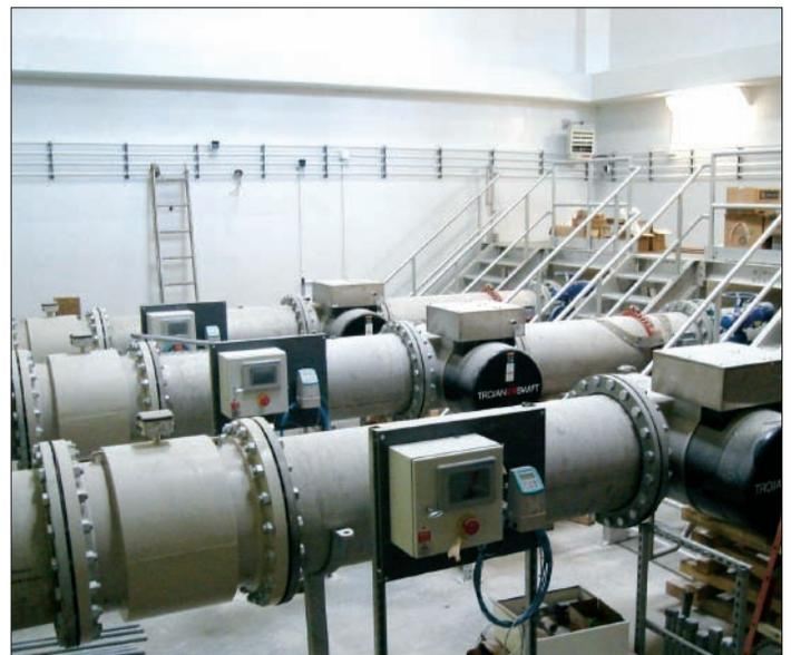
Figure 5. shows the UV Building process area
