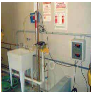
Figure 4: Setup for the UV disinfection pilot study at Norfolk, MA .
